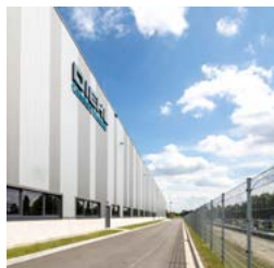
Hamburg Interlink Logistics Centre
